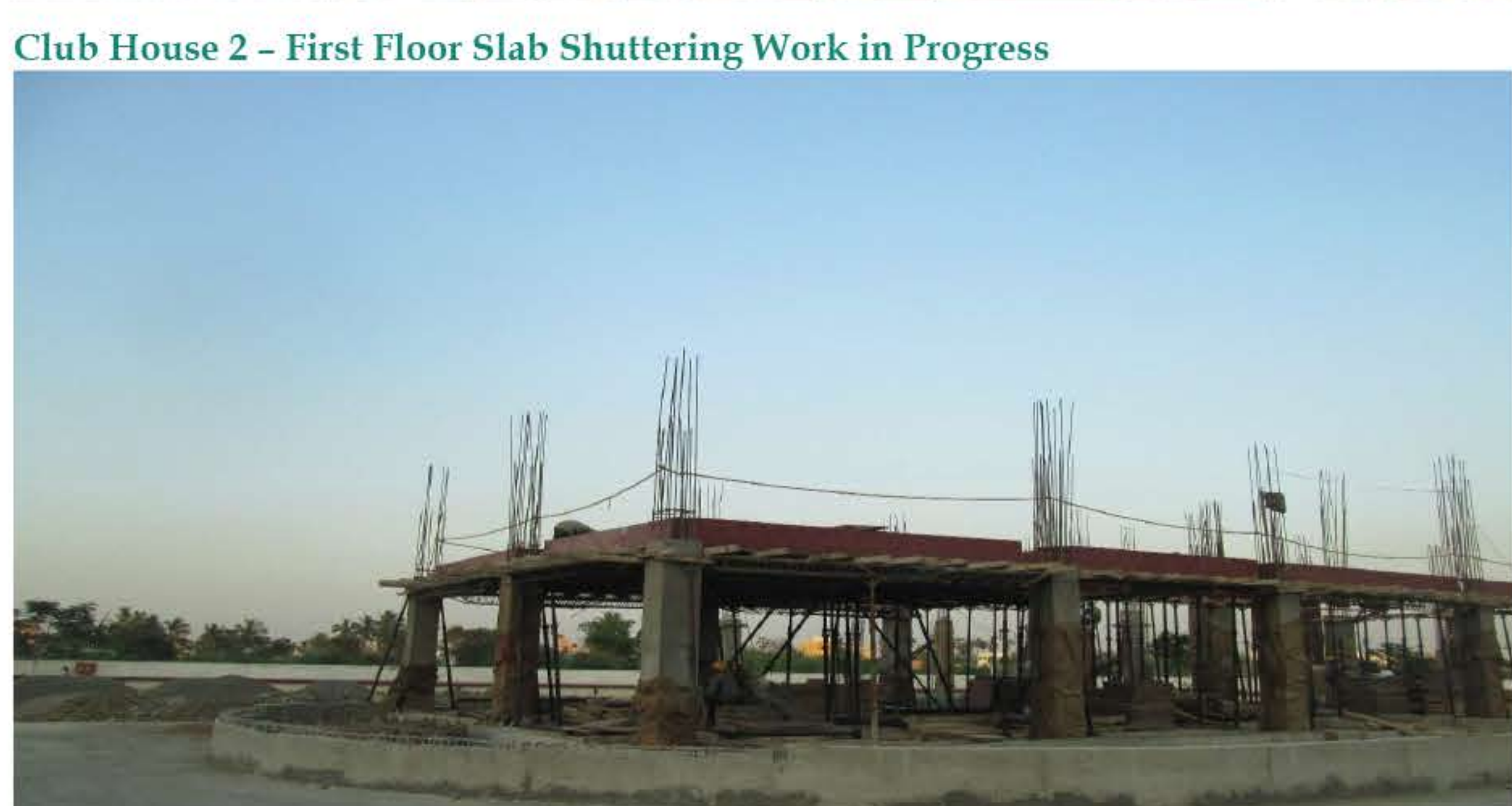
Club House 2 - First Floor Slab Shuttering Work in Progress
