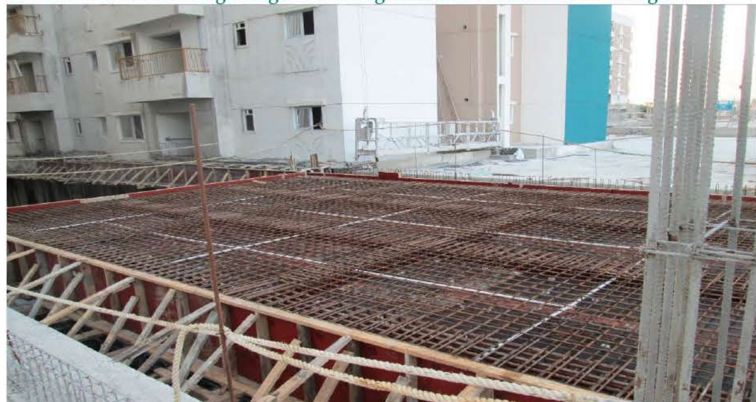
Club House 2 - First Floor Slab Shuttering Work in Progress
