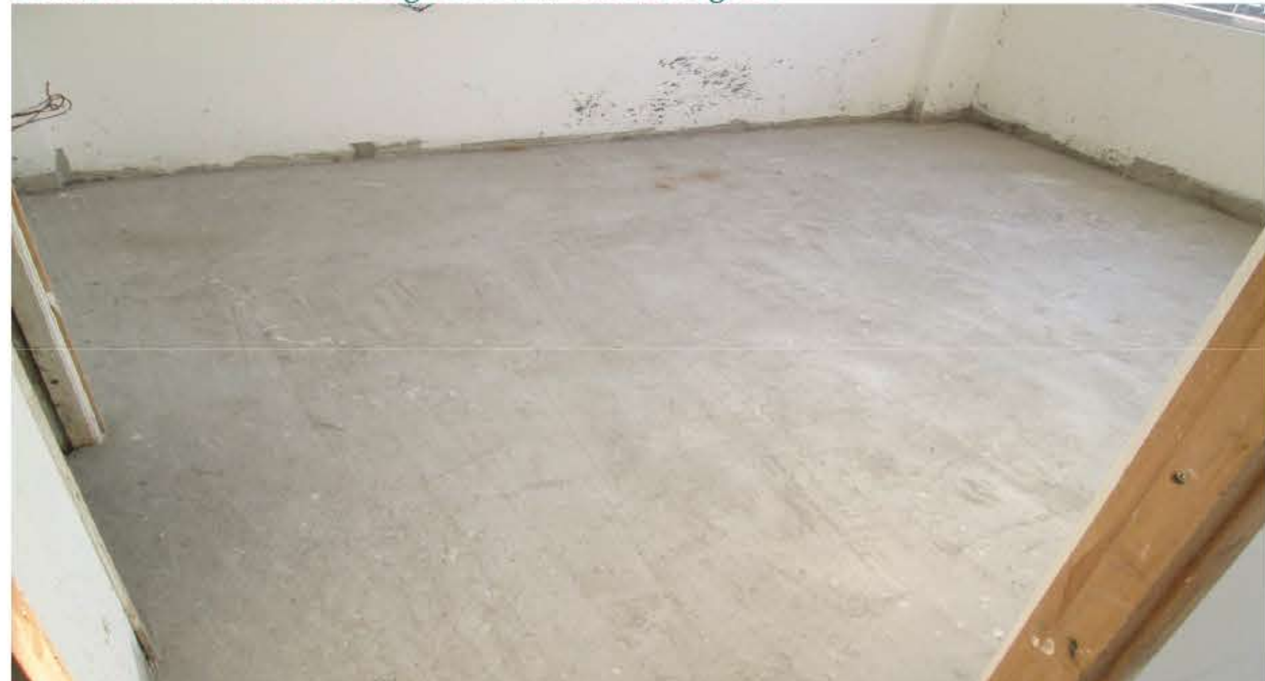
Tower H - Wooden Flooring Screed Work in Progress
