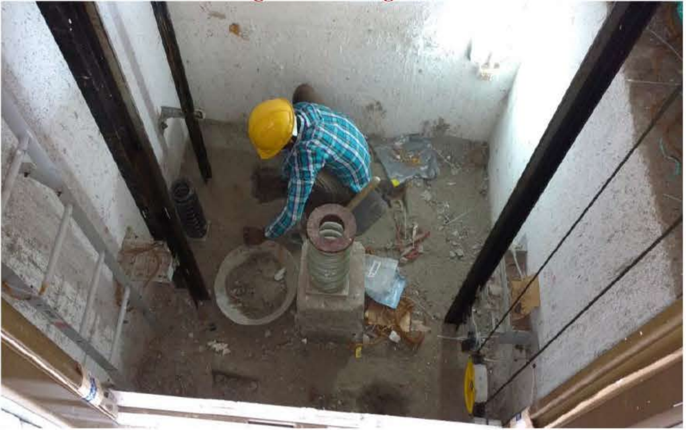
CH - Lift Pit Inner Cleaning Work in Progress.
