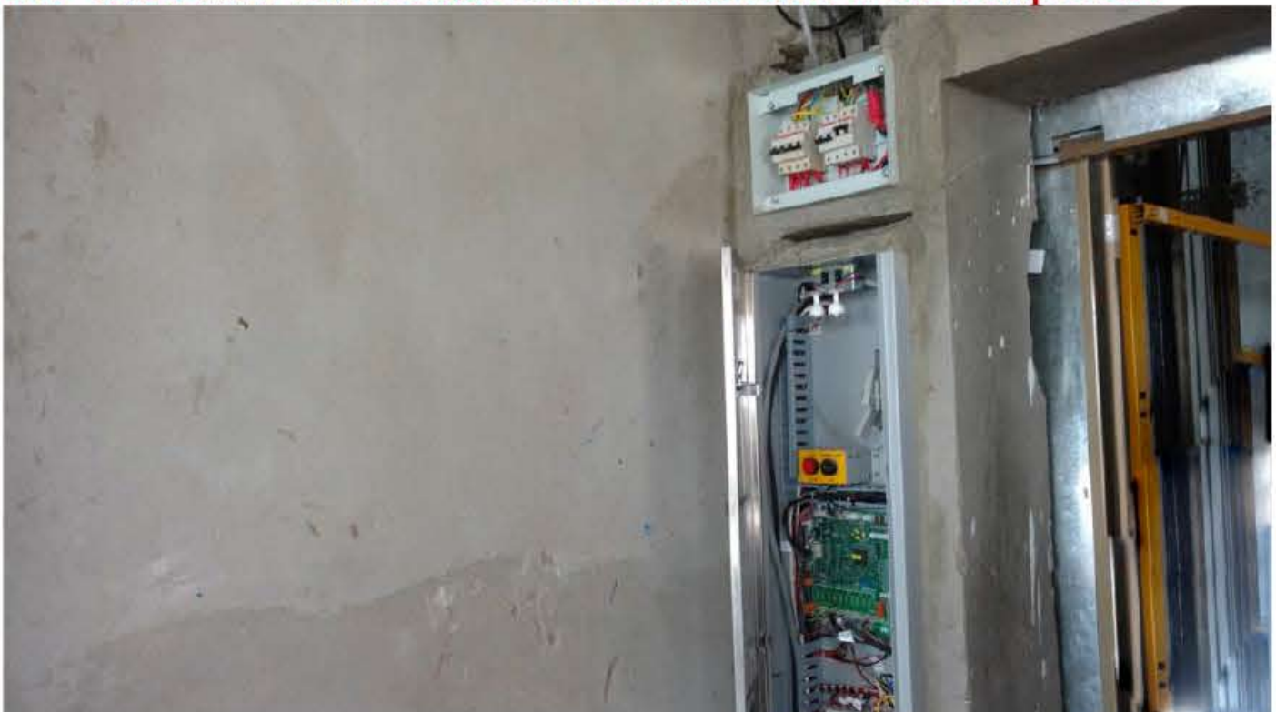
CH - FIRE LIFT Three Phase Power Connection Work Completed .
